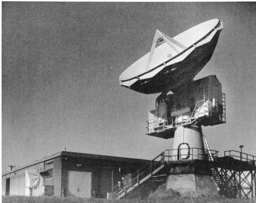
FIG. 18.1 AN/FPQ-6 C-band monopulse precision tracking radar installation at the NASA Wallops Island Station, Va. It has a 29-ft-diameter antenna and a specified angle precision of 0.05 mrad rms.
